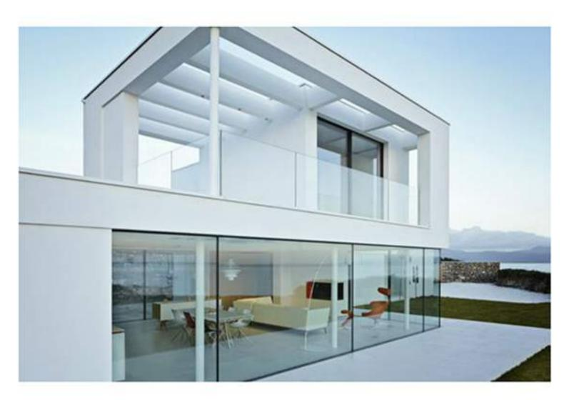
o what is structural glazing? In short it's where glass becomes an intrinsic part of the structure, where its load-bearing capabilities are as, if not more, important than its' aesthetic appeal.
